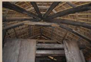
Fig. Roofing system in Khasi house
